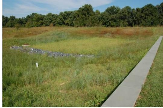
Similarly, the yard area around Darlington Hall has 3 micro-bioretenion facilities plus an installation of pervious pavement on the south side. The micro-bioretenion cells are carefully graded into the landscape close to the architecture and, in some cases, sculpted into narrow spaces between the building and the Thomas Run Road right-of-way. The permeable pavement is installed along a pedestrian pathway connecting the main building entrance with parking lot "C."
